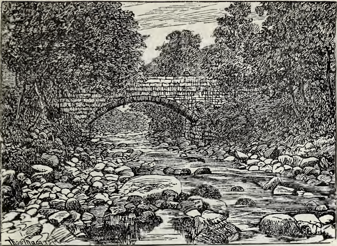
Bridge over How Stean Beck.
